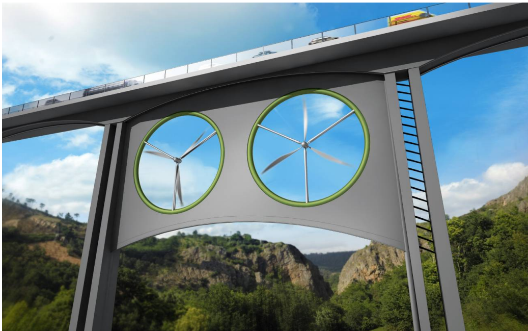
Illustration of two identical wind turbines installed in a viaduct. / José Antonio Peñas (Sinc)
